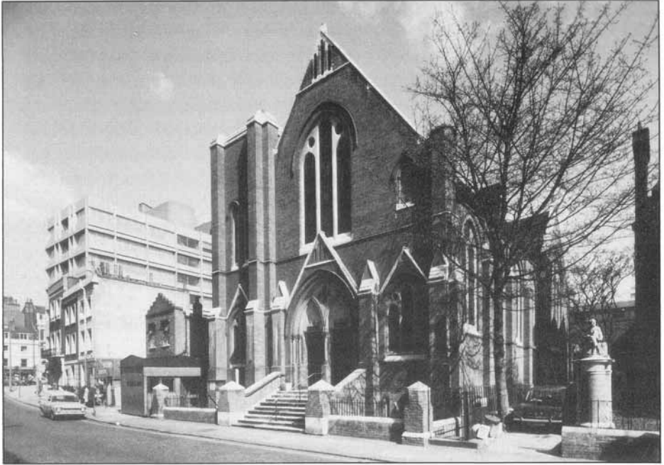
The Church just prior to demolition in 1973; the spire had been removed in 1960. Note the 'Boy Monument' to the right. (NMR BB73/2456).
