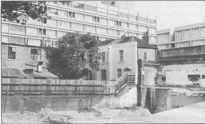
The 'Hole in the Ground', Essex Church 1973/77. The Czech Embassy fills the background in this September 1973 photograph (RBK&C Local Studies Library KE 73/338).
